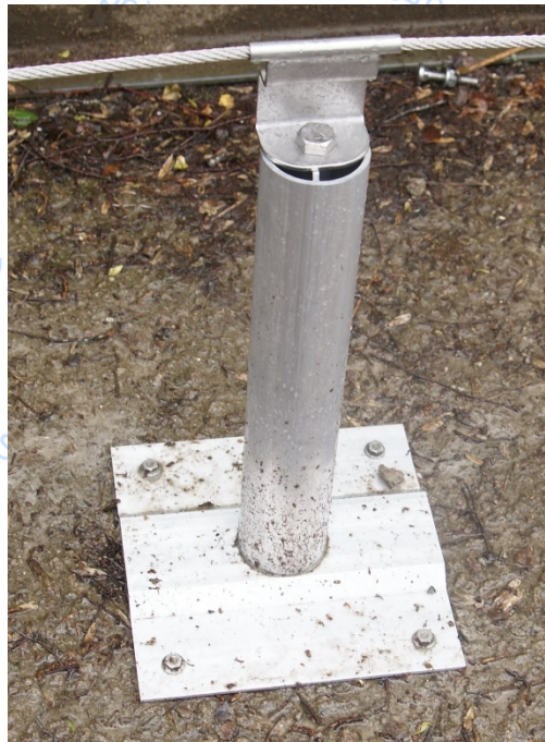
Figure 2 – Intermediate anchor from horizontal anchor described as “FSL.0270.0450.3U”
