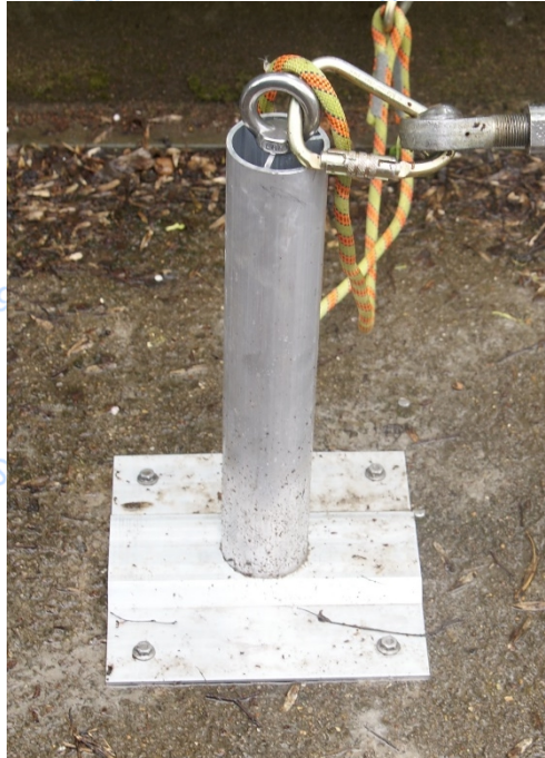
Figure 1 – End anchor from horizontal anchor described as “FSL.0270.0450.3U”
